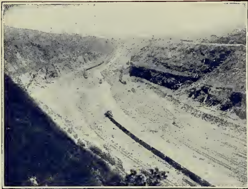
The Completed Gaillard Cut at Empire, Looking North
